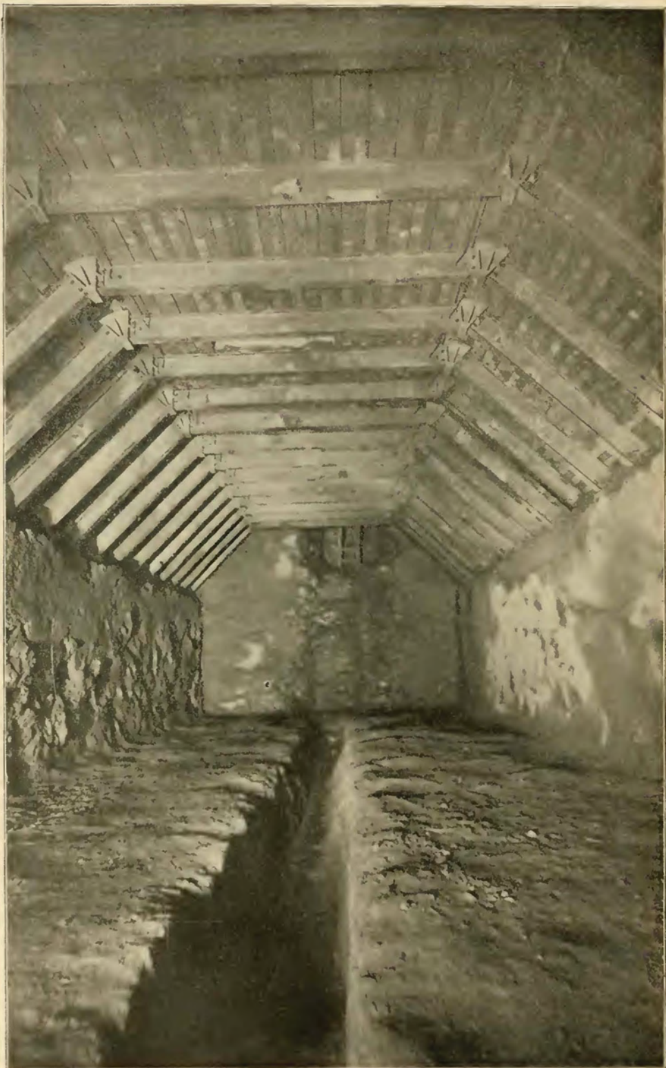
Pump House, Hazleton Shaft Colliery.
