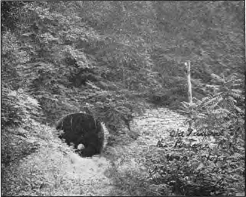
ALLEGHENY PORTAGE TUNNEL, 1834. Eastern Opening.
