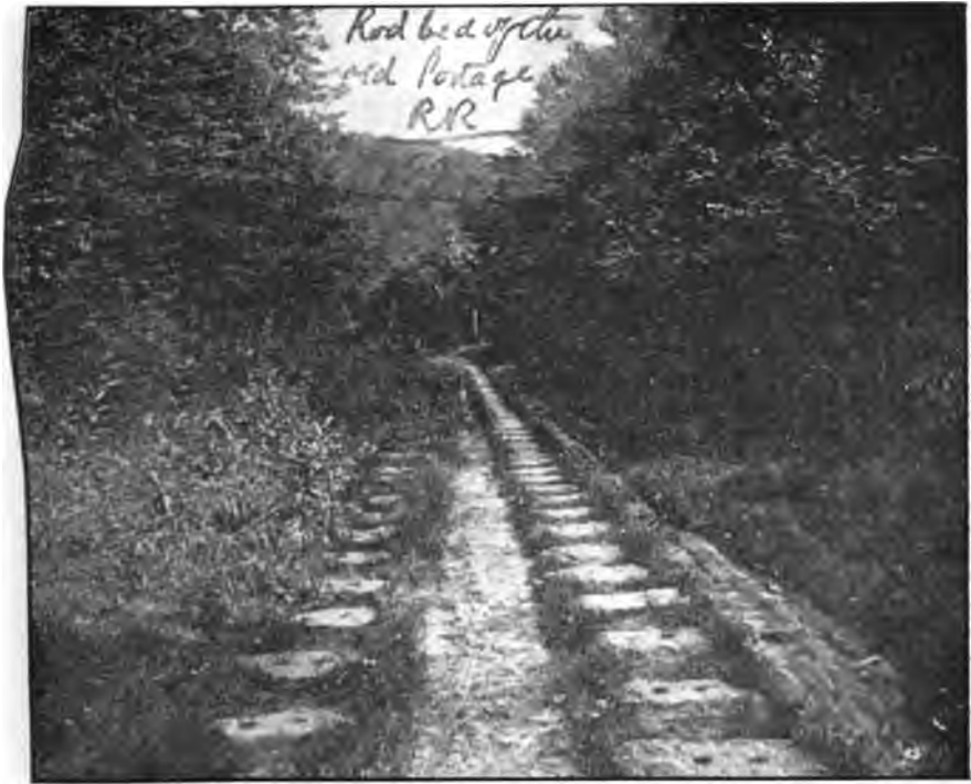
RUINS OF OLD PORTAGE ROADBED. West of Plane 8.
