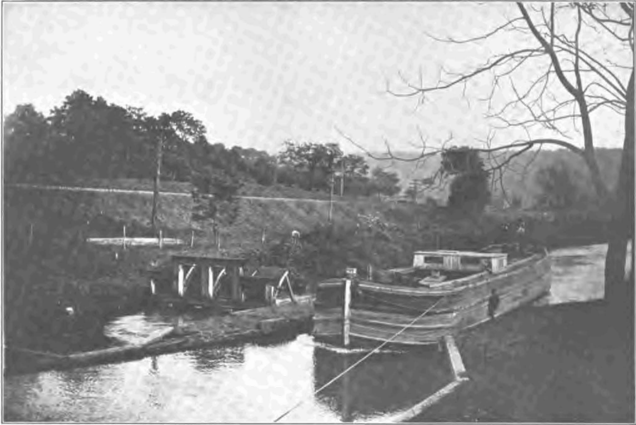
Canal Guard Lock, Dauphin Narrows used to check the current of the river, when at flood stage and flowing into Canal.
