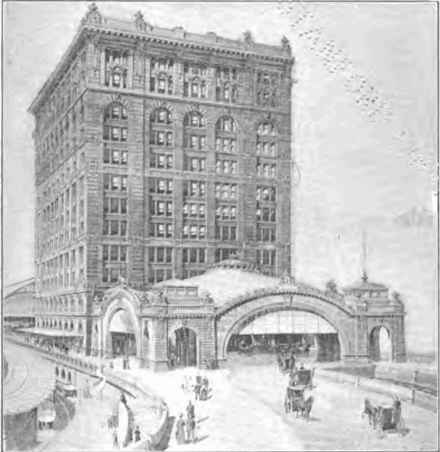
NEW UNION STATION, PITTSBURG, PA. Pennsylvania Railroad Company.
